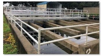
through the chlorine contact basin, where the chlorine has time to meet the demand needed before distribution.
